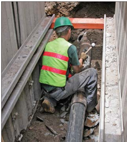
Above, the electrofusion coupling process is used to join the final joint and connect the new pipe to the valve assembly. Below, detaching the bursting head in the middle pit.
