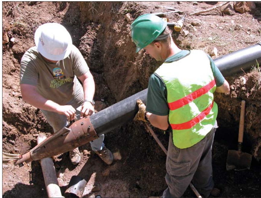
Final adjustments are made to the pipe attachment.
