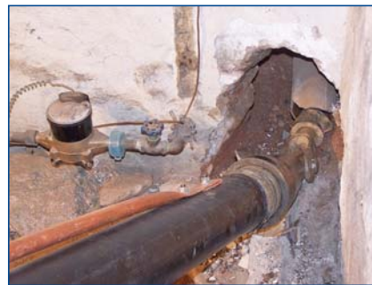
A section of HDPE pipe ready to pull ...
